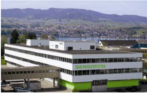
Sensirion headquarters in Staefa, Switzerland
